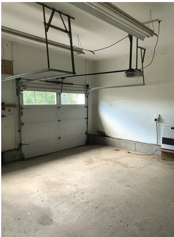
Both garage doors were removed and “dummy” doors re-created outside (even fooling the snow-plow guy!)
